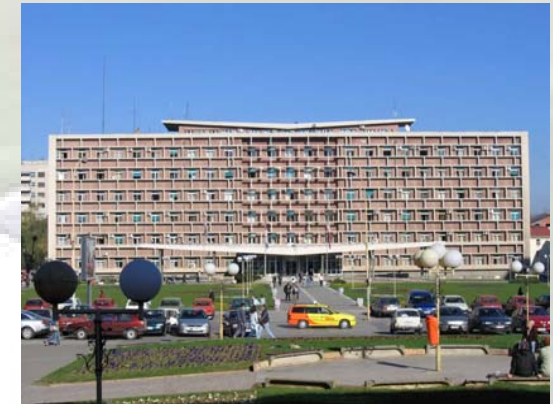
City Hall of Kragujevac
